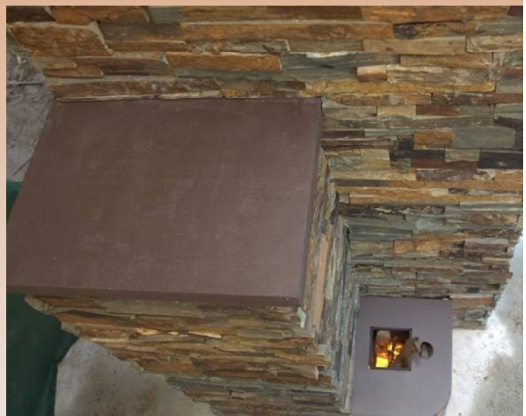
The short columns are the combustion system and the tall columns are the heat storage chambers.
