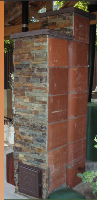
Flues used to build Heat Storage Chambers
